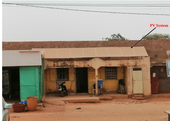
Fig. 3. PV system in roofing of shop in Ouagadougou City
