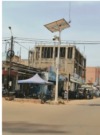
Fig. 1. Surveillance camera powered by PV energy to control road traffic in the City of Ouagadougou (Burkina Faso)
