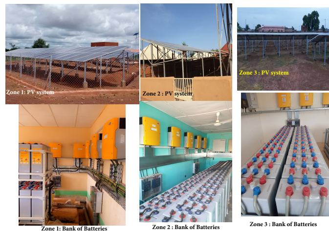
Fig. 6. 50kW_p power plant installed in the three climatic zones of Burkina Faso
