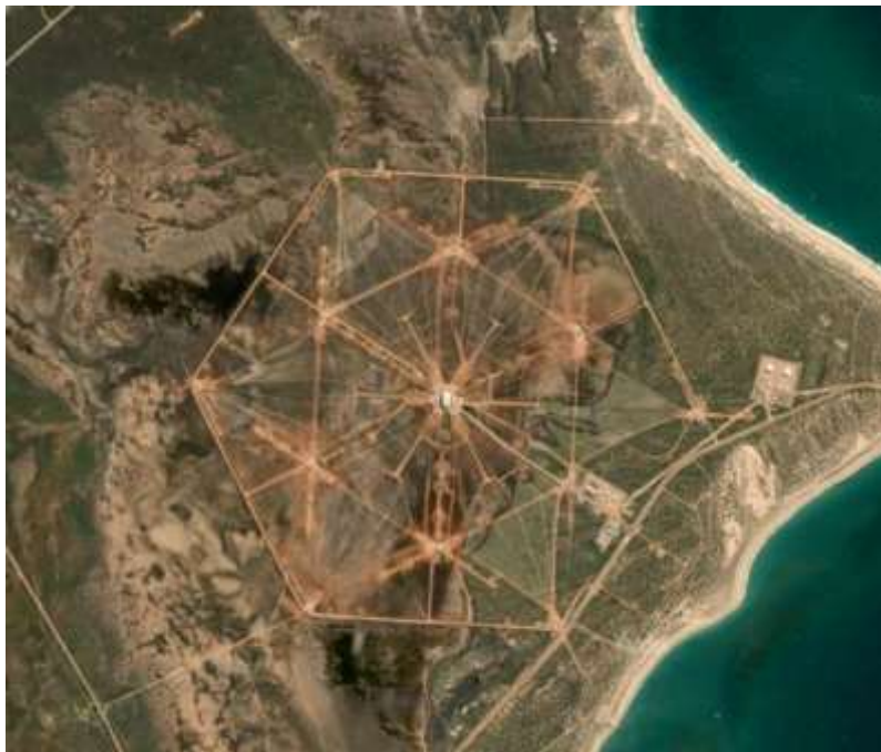
Fig. 3. Australia, powerful VLF transmitter (North West Cape (NWC) transmitter: Naval Communication Station Harold E. Holt) [45]
