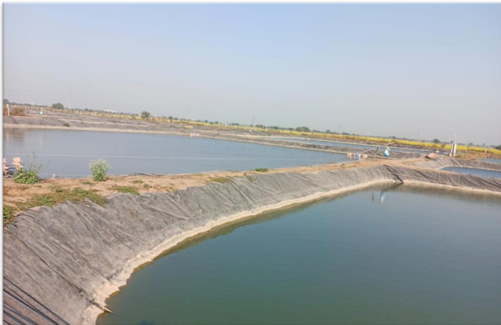
Fig. 5. Geomembrane-covered ponds ponds at Jhanjarola, Gurugram, Haryana
