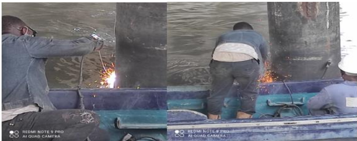
Fig. 4. Images of welding exercise of the anodes on the casing pipes
