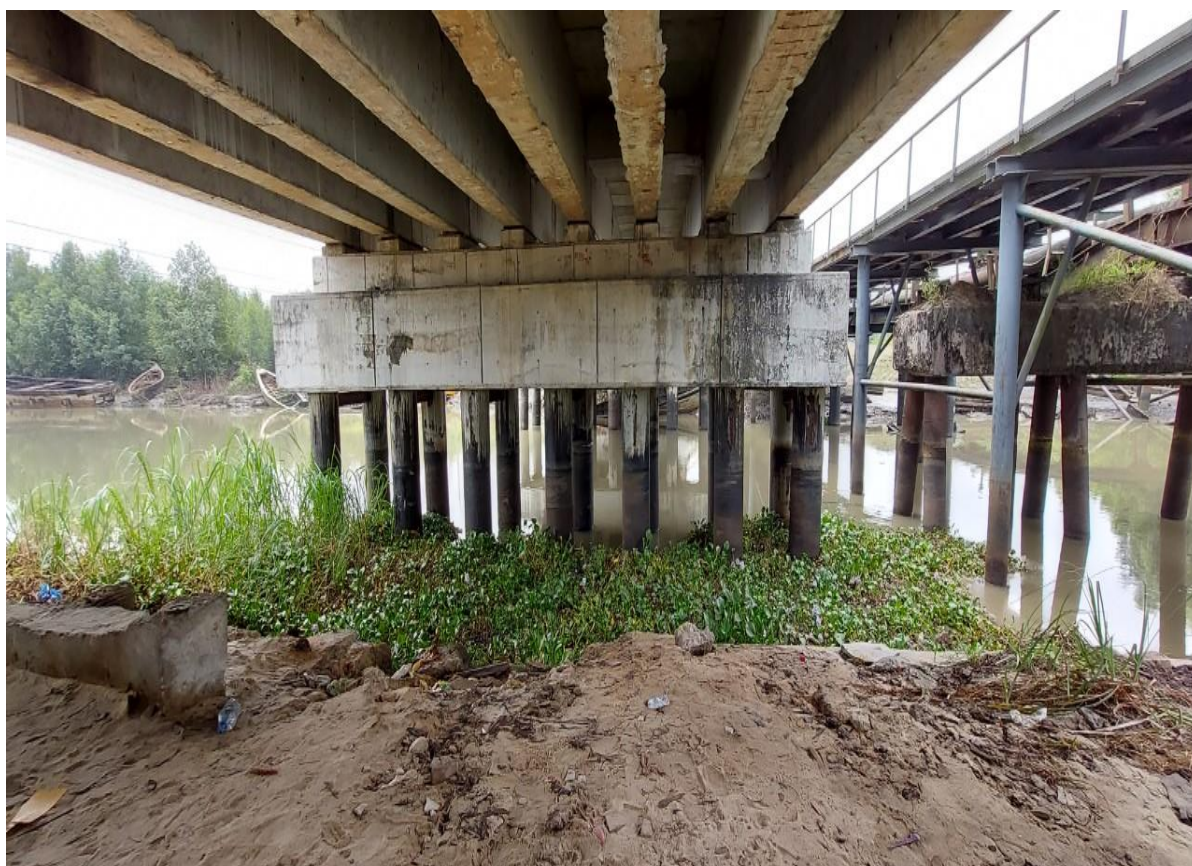
Fig. 1. Image of the 60 m reinforced concrete bridge structure
