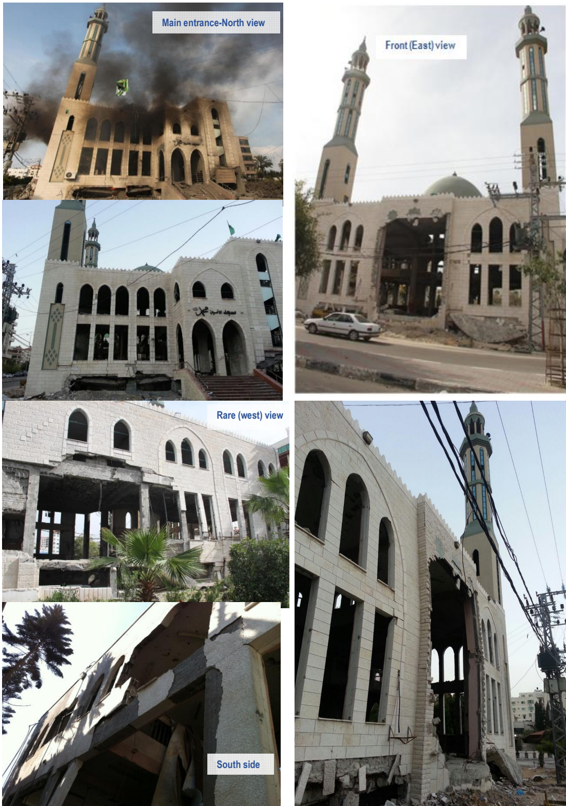
Fig. 2. Damage to Al-Amin Mosque- outside photos
