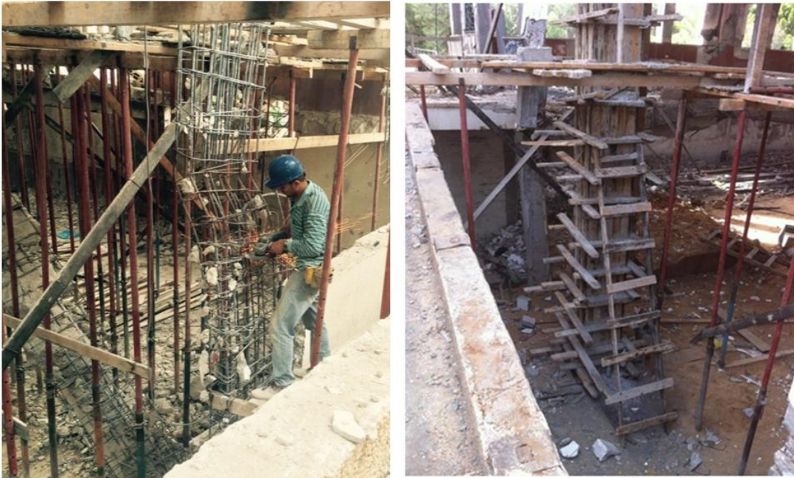
Fig. 5. Replacing damaged columns
